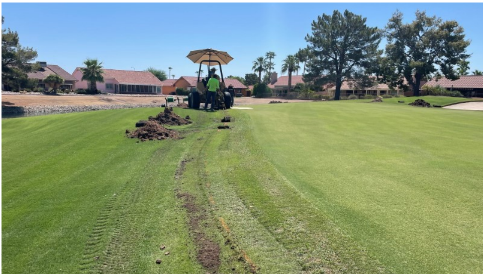
Pulling wire around a green on Grandview leaves little disruption and the recovery time is minimal.
